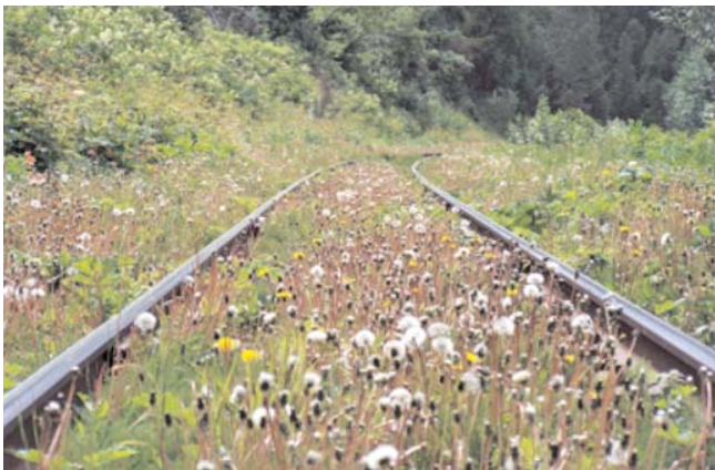
Overgrown weeds on the track bed are nearly impossible to eliminate with non-chemical methods.
