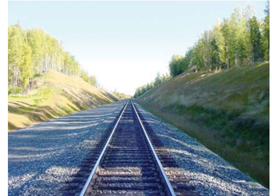
Newly-laid track ballast does not require vegetation control for a few years.
