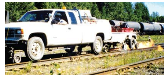
Burning and hot water/steam have met with little success as alternative vegetation control methods.
