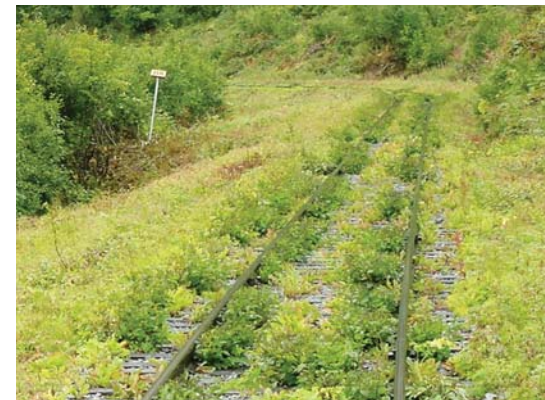
The ARRC right-of-way can provide a vector for the spread of invasive, noxious weeds.
