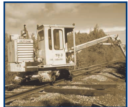
The railroad replaces more than 100,000 ties a year.
