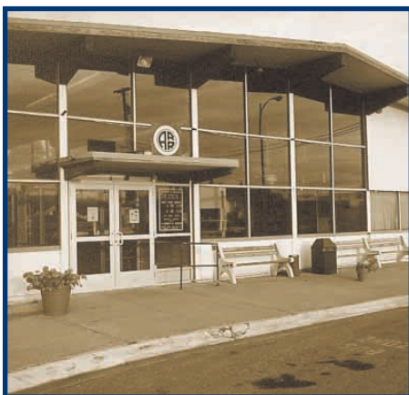
Fairbanks has outgrown the existing depot.
