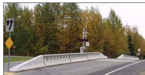
Median barriers at Oceanview Rd crossing.
