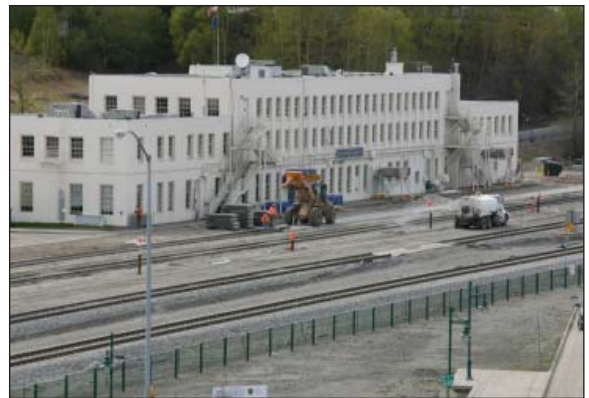
Anchorage Historic Depot track work in 2009.
