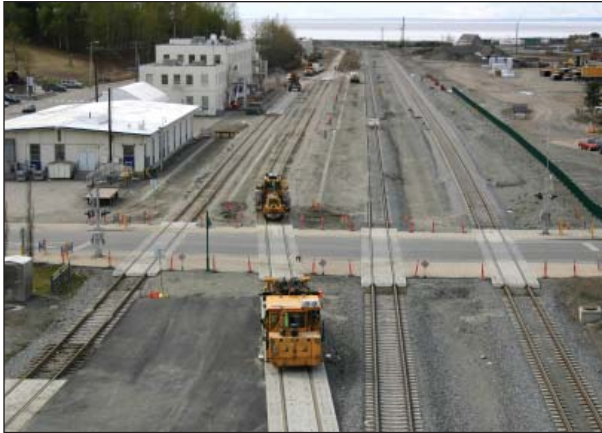
Phase 1 added tracks and was complete by fall 2009.
