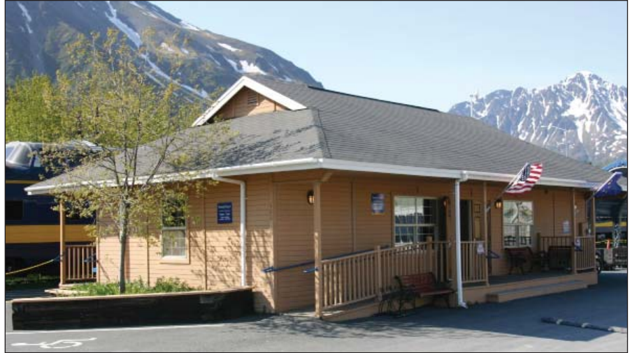
The Seward Depot May 2009. The ramp and stairs will be similar for the restroom facility.
