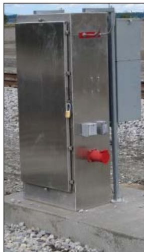
The Shore Power cabinet will be similar to the one in the Anchorage yard (pictured).
