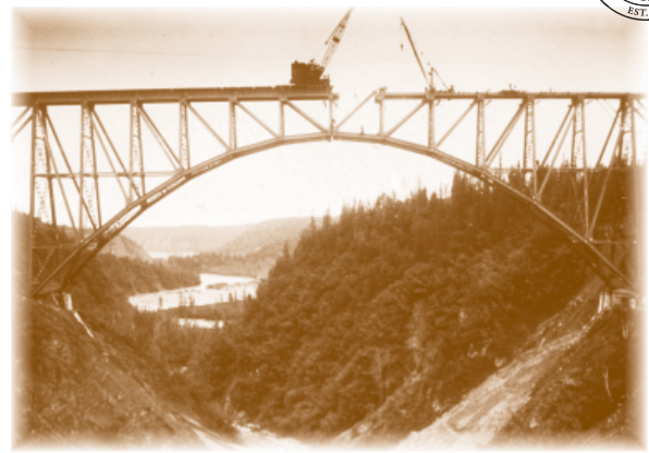
Built in 1921, the 914-foot Hurricane Gulch Bridge at Milepost 284.2 is a remarkable feat of engineering. It is eligible for the National Register of Historical Places. This photo of this iconic bridge is part of the Alaska Railroad's collection of historic photos archived at the Anchorage Museum of History and Art.
