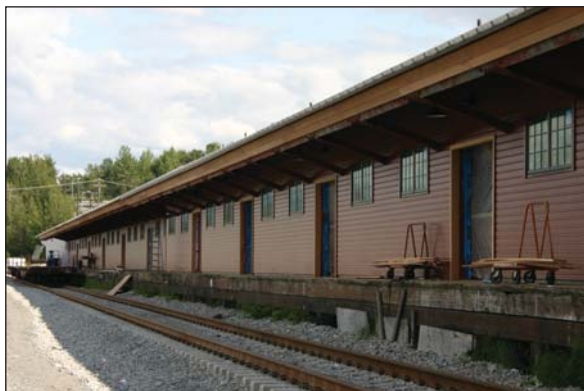
New siding gives the shed's back side a facelift.
