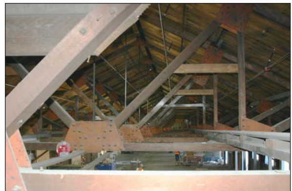
Large-timber rafters remain as a prominent interior feature.
