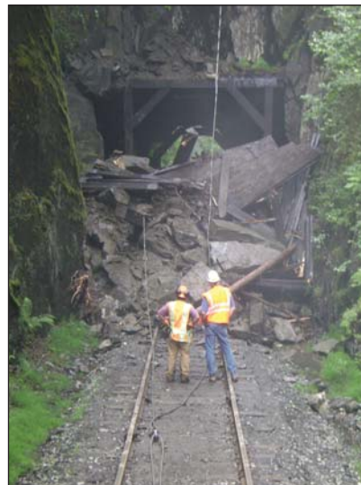
A July 2009 rock slide temporarily closed access through the tunnel about 50 miles north of Seward. A new “rock shed” will be installed to protect trains from falling rocks and ice.
