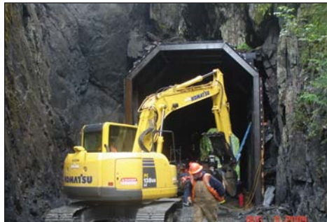
A July 2009 rock slide temporarily closed access through the tunnel about 50 miles north of Seward. A new “rock shed” will be installed to protect trains from falling rocks and ice.
