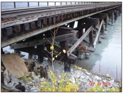
Steel will replace much of the timber on Bridge 29.5 (Moose Pass).
