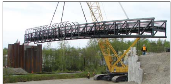
Below right: Crews place the pedestrian bridge June 2008.
