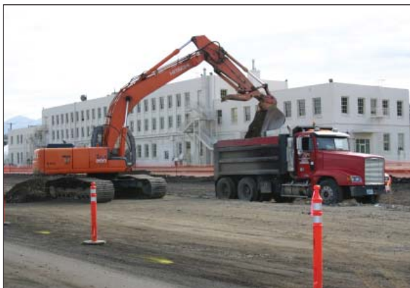
Earth work for additional tracks got underway in 2007.
